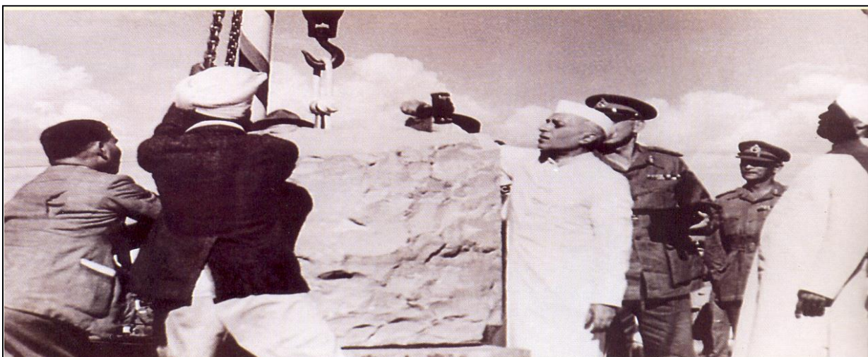
"A MONUMENT IN THE MAKING" – PANDIT JAWAHARLAL NEHRU, THE HON'BLE PM OF INDIA, LAYING THE FOUNDATION STONE AT KHADAKWASLA ON 06 OCT 1949
